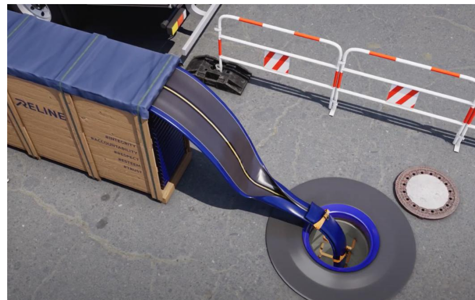
Figure 3: The liner is taken from the transport box and inserted in the gravity sewer or stormwater pipe © RelineEurope GmbH
