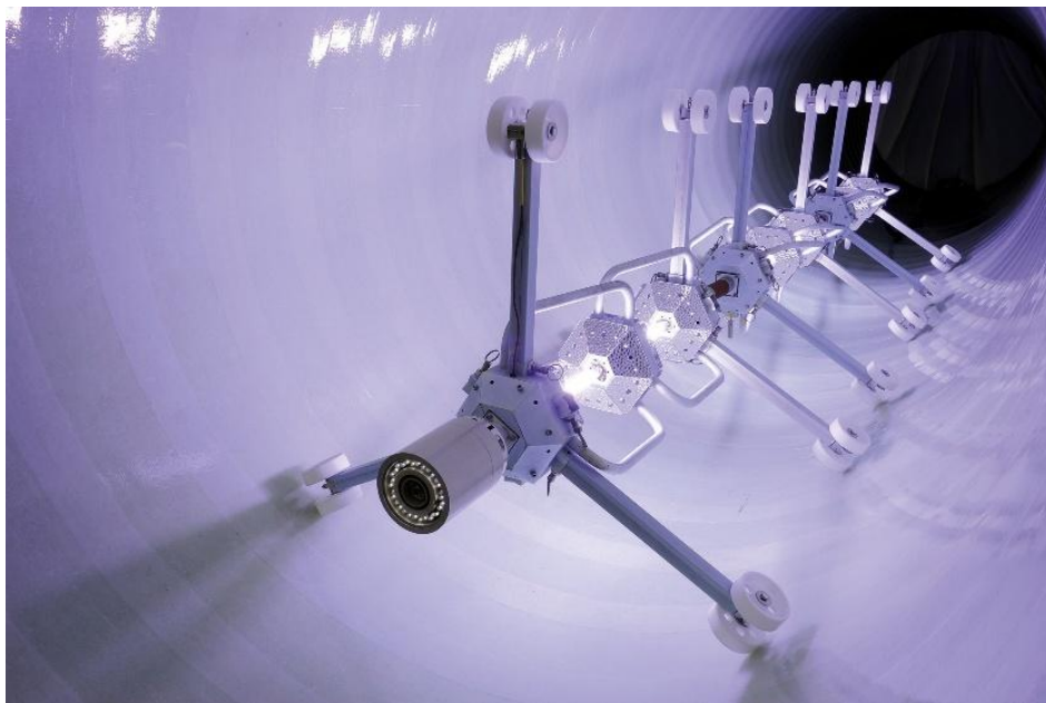
Figure 4: Inside view of a liner during curing with UV light. © RelineEurope GmbH
